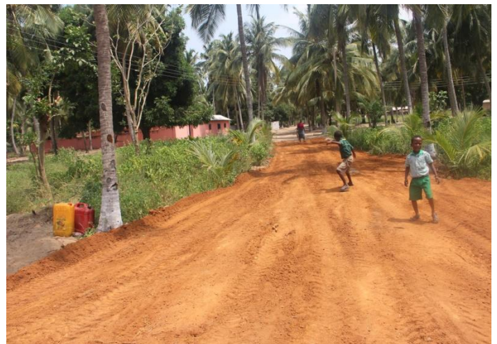
Road to Worgbato after construction
