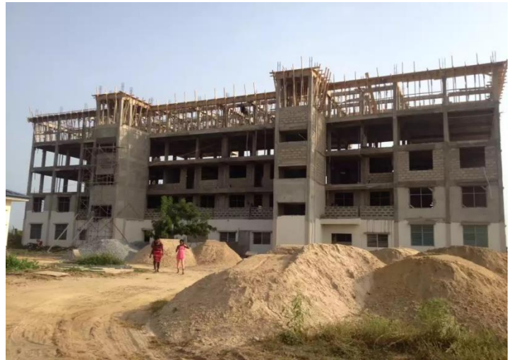
Staff apartments under construction
