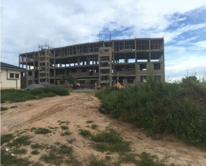
Staff apartments under construction
