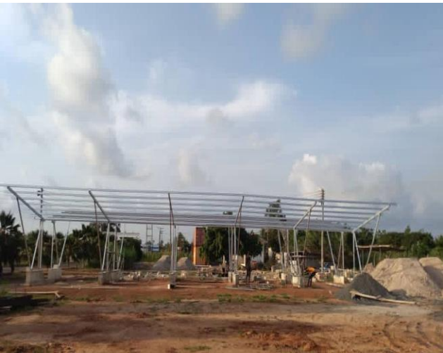
Hospital Solar Power System Under construction
