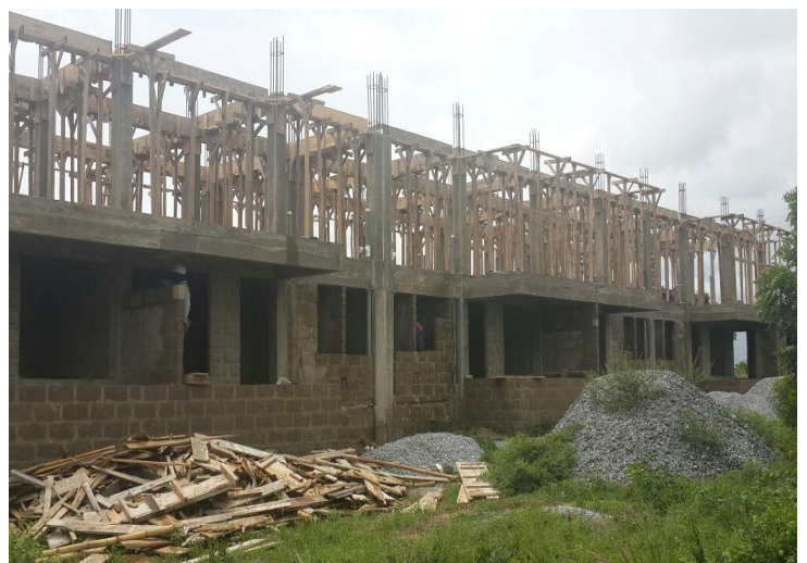
Staff apartments under construction
