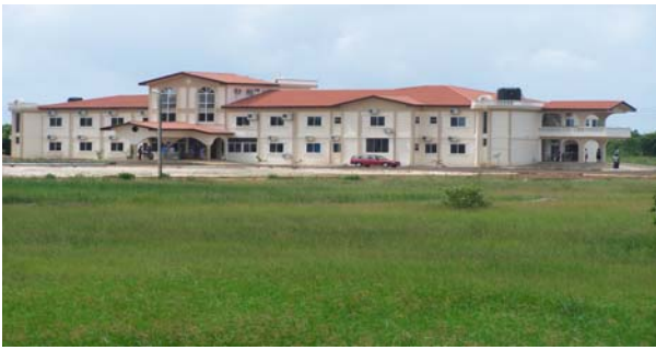
Front View of Hospital
