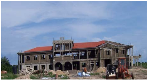
Front view of the Outpatient building with new roofing
