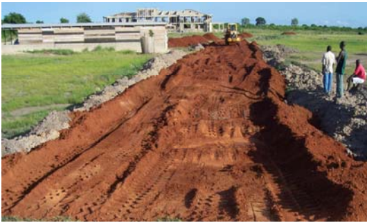
Driveway under construction
