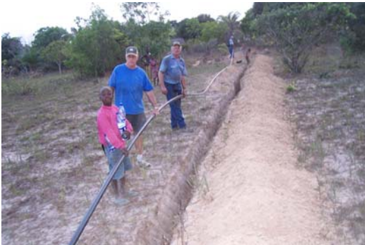
Dave & Dale working on pipeline
