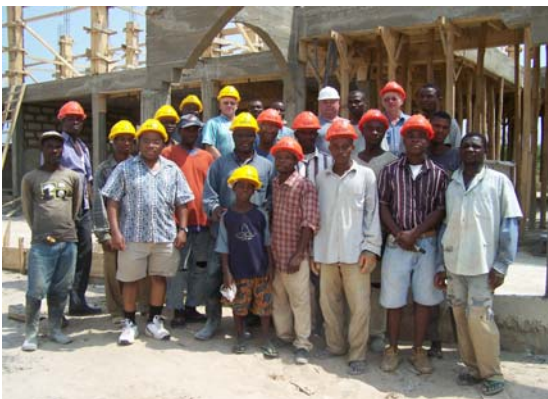
Ghanaian construction team with part of team
