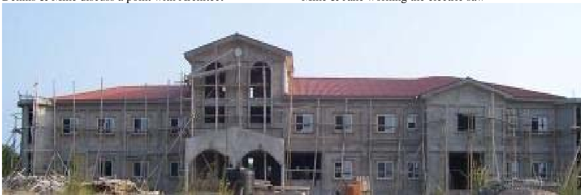
Front view of outpatient clinic building currently under construction
