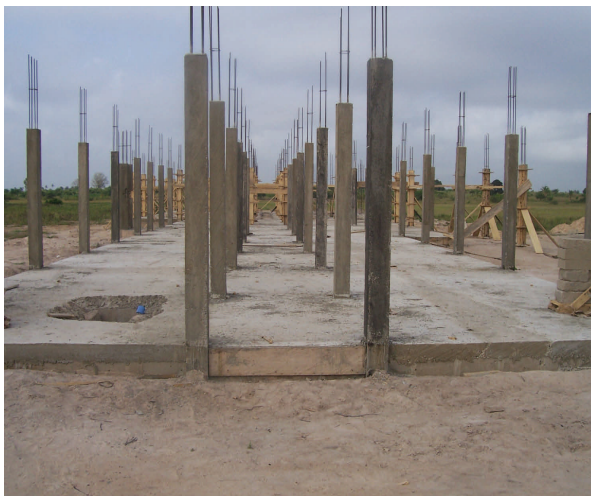
Foundation completed, Columns up—Nov 27, 2006
