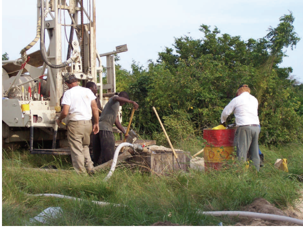
Unsuccessful drilling for water - Sep 29, 2006
