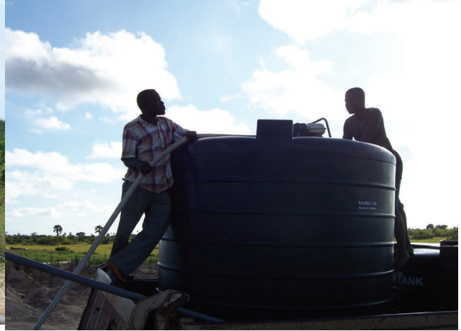
Delivering of water at Construction project site -Oct 21,
