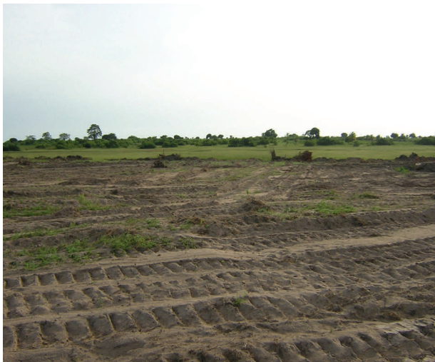
Site Preparation for IHDN Hospital - June 10, 2006
