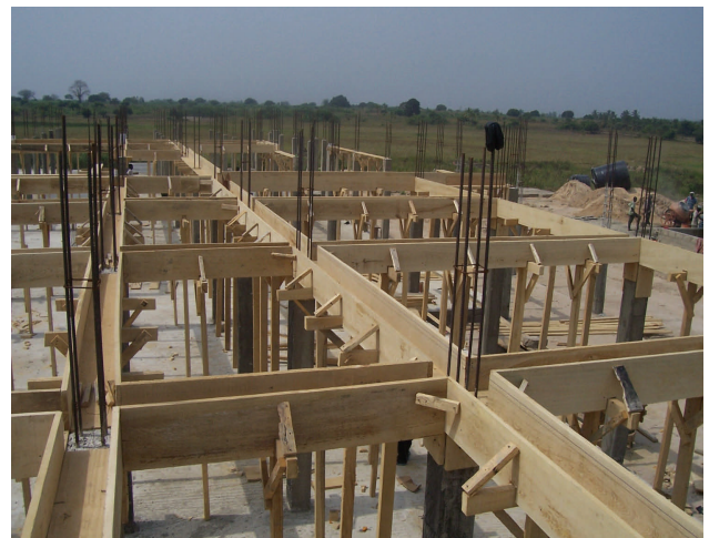
Construction of Beams - December 10, 2006
