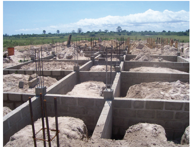
Foundation work in progress— October 16, 2006
