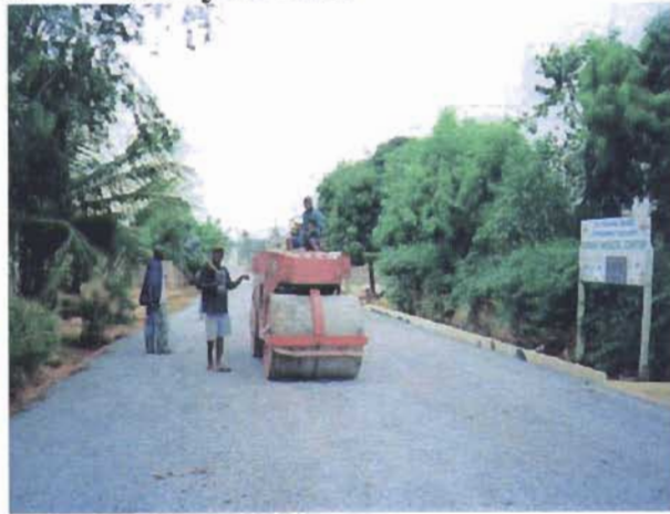
Road Construction in Ghana - 2003
