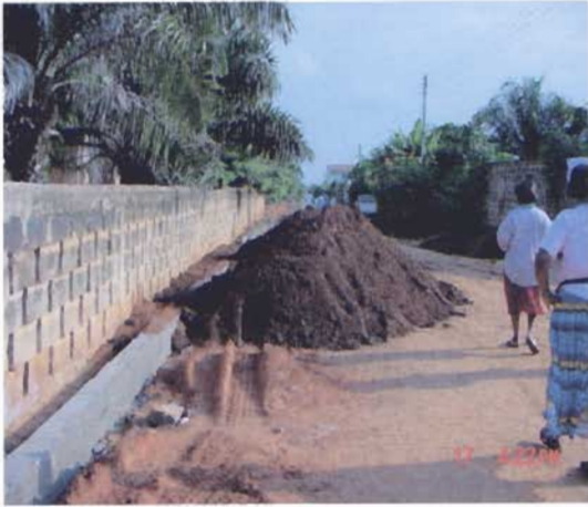
Road Construction in Ghana – 2002
